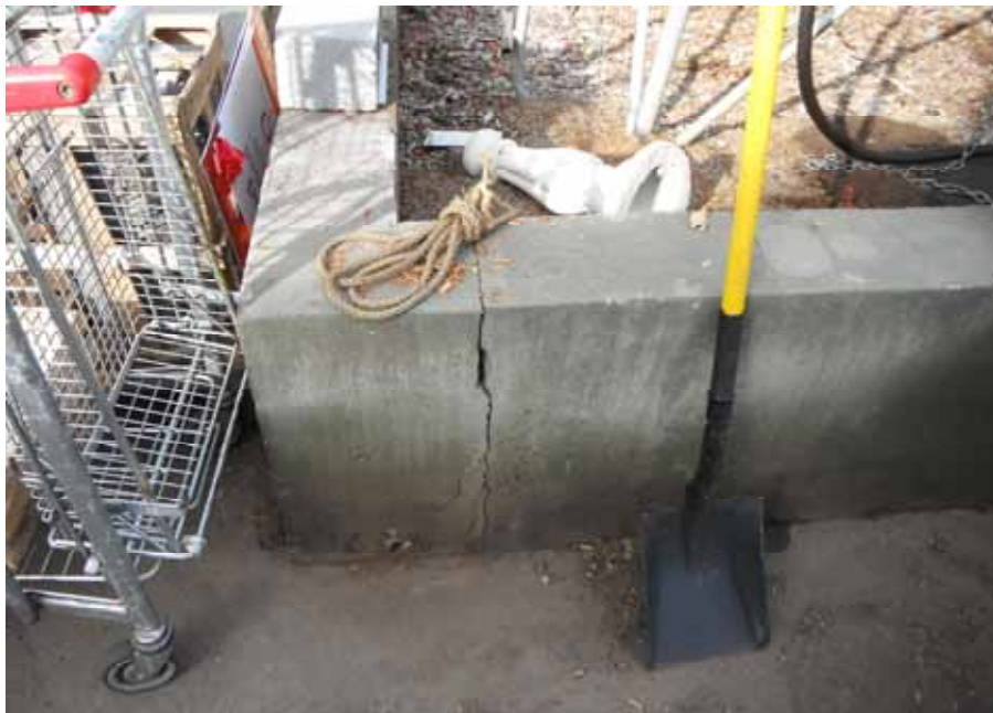
Photo 10 – Cracks in fuel tank bund
