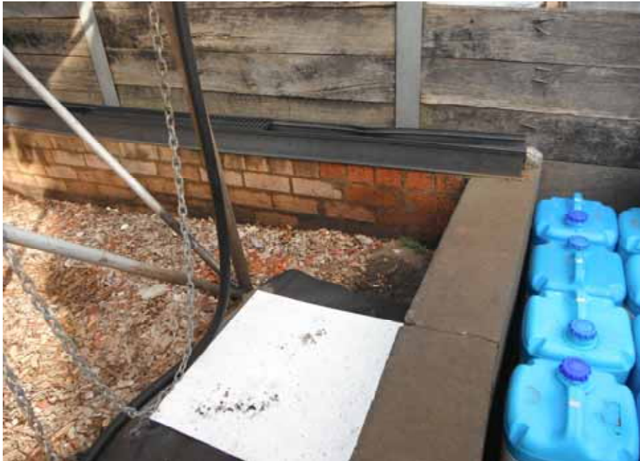
Photo 11– Brick lining of bund and further cracks
